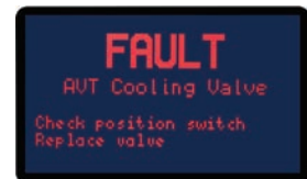
AVT Valve Fault Screen.
