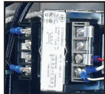
Control circuit transformer fuse
