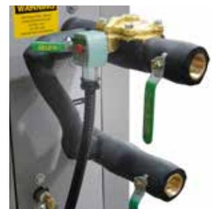
**C. PROCESS LINE SHUT OFF VALVES:** These valves are full size ball valves installed on the “to” and “from” process lines at the exit of the chiller. These valves can be used to adjust the process flow rate and to shut off the flow rate to isolate the chiller.
