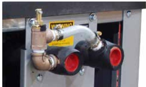
Typical Automatic Low Flow Bypass Valve
