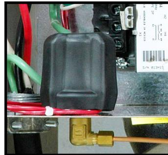
Panel mounted pressure switch Figure 3.2A
