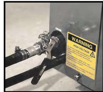
Typical drain valve installation
