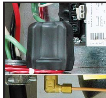
Panel mounted pressure switch Figure 3.2A
