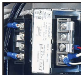
Typical control circuit transformer fuse
